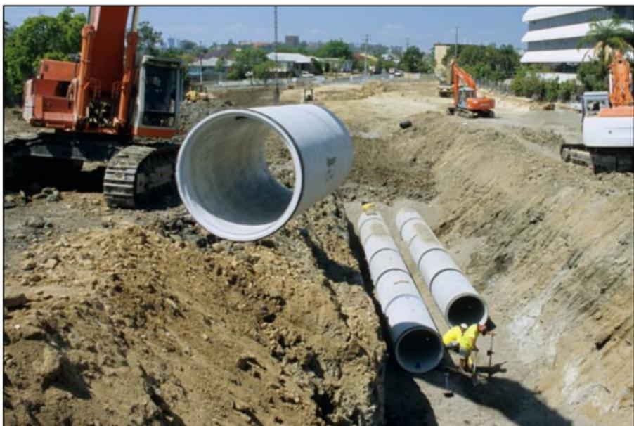
*Example of a good installation - trenches are neatly excavated and the pipes are progressively backfilled.*
