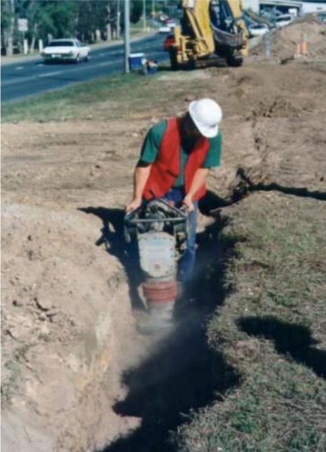
*Initial backfill compaction being undertaken with a hand held compactor - a controlled operation.*
