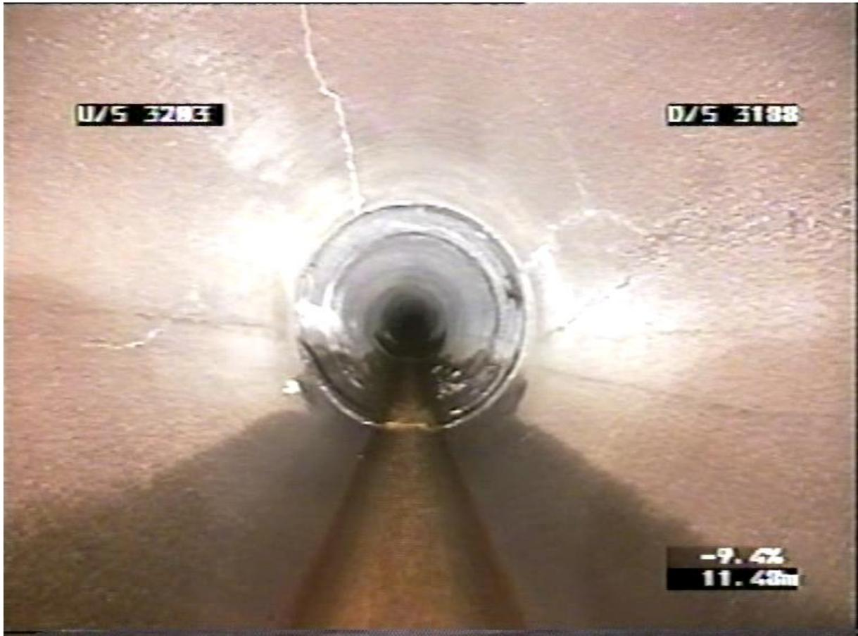
In the second photograph the cracking is a little wider but appears to have autogenously healed. A prudent engineer would confirm this scenario.
