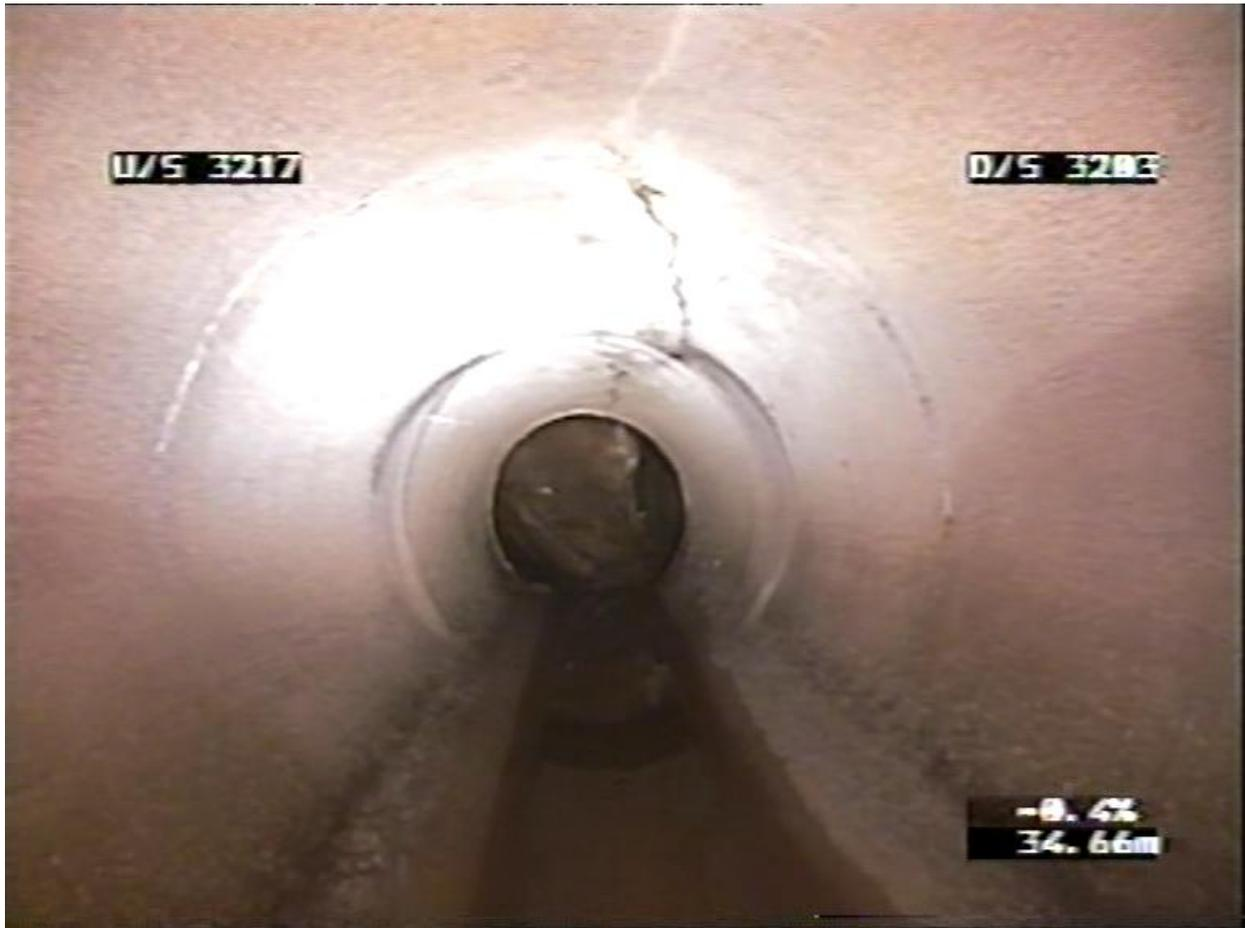
This pipe was well within design depth and had no superimposed load. It is assumed that the crack at 12 o'clock and the apparent deformation was caused by temporary earthmoving loads.
