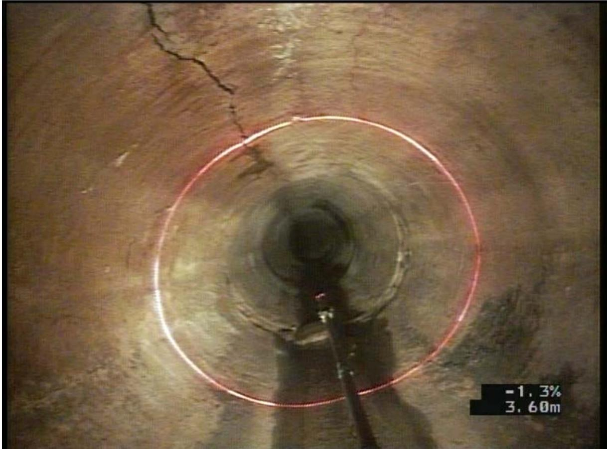
This photograph was taken during laser profiling of a concrete stormwater about 1500mm diameter. The laser light provides an indication of the extent of the deformation of the pipeline.
