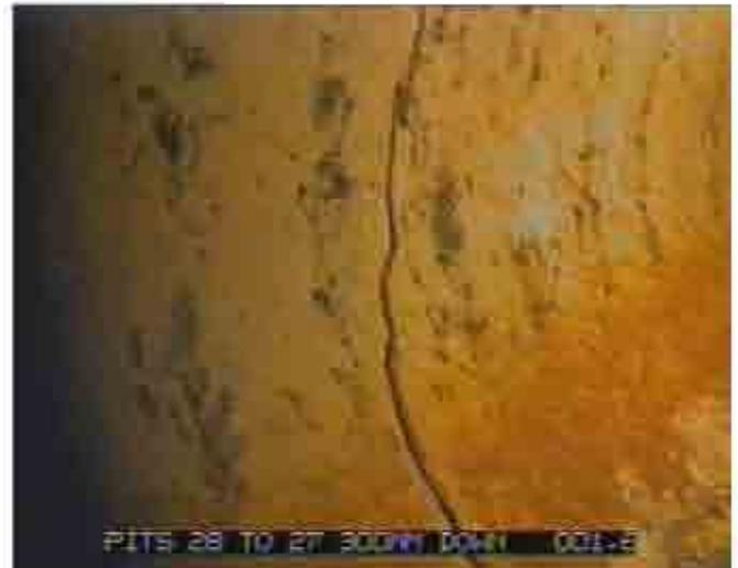
*An internal circumferential crack of a DN300 concrete pipe, greater than 0.5mm wide.*
