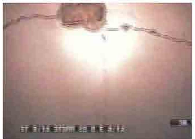
*An internal circumferential crack of a DN375 concrete pipe, greater than 0.5mm wide.*
